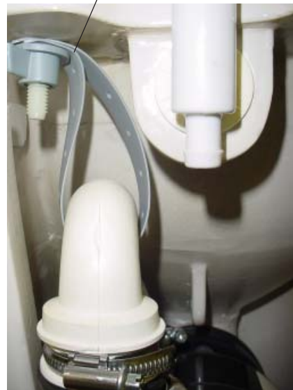
Fig. 19A Discharge support strap
